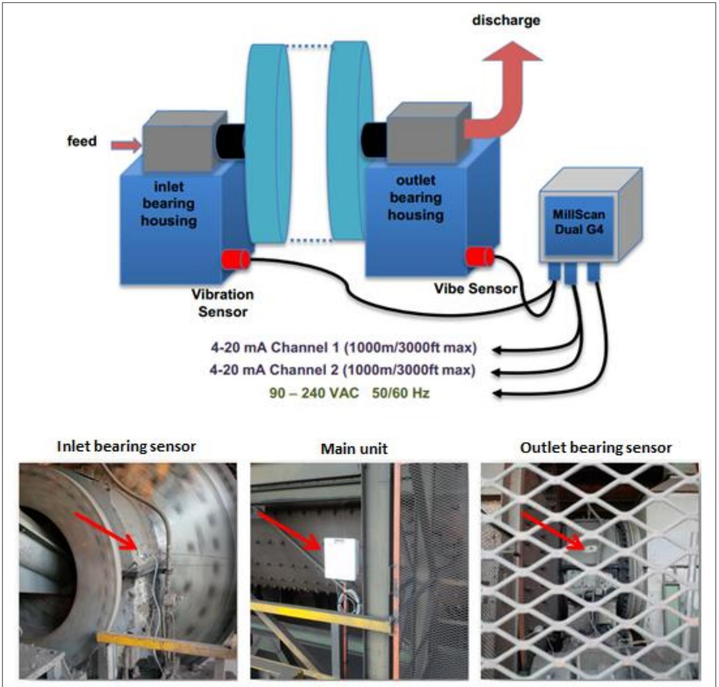
Figure 2-1: MillScan G4 components and configuration (Images taken at Xstrata Lion Mill B).
